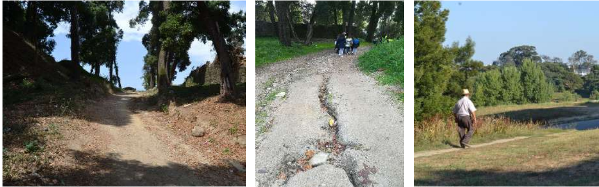
Figure 27. Precarious conditions found along the current paths.
