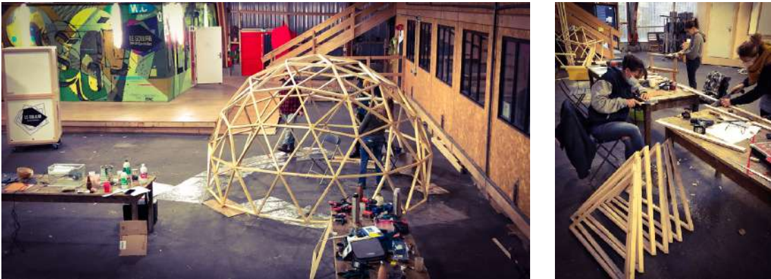
Figure 33. Prefabrication of the greenhouse in the association's workshop (Source: Association Bio-T-Full).
