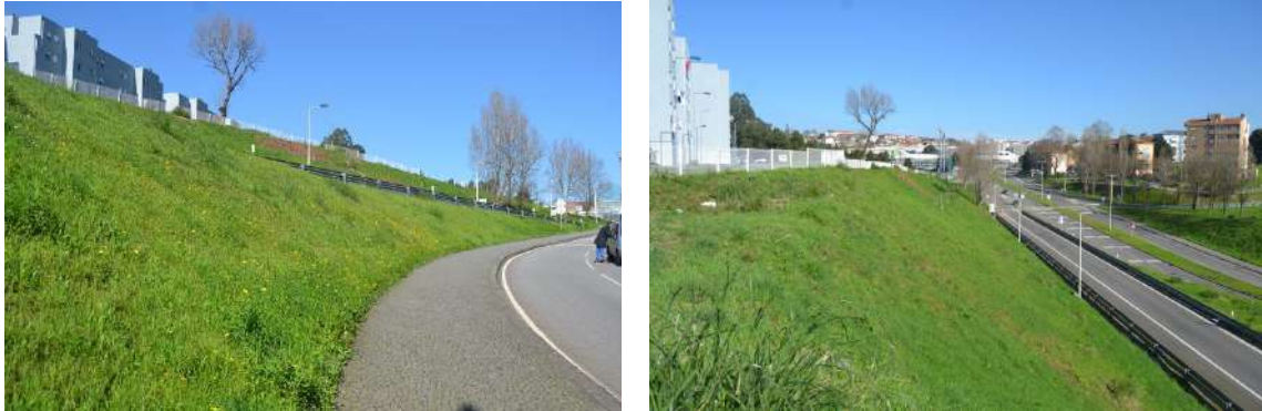
Figure 47. Large slopes next to Avenida Artur de Andrade
