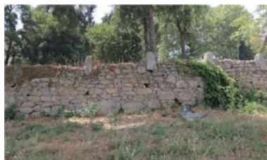
— Granite masonry walls
