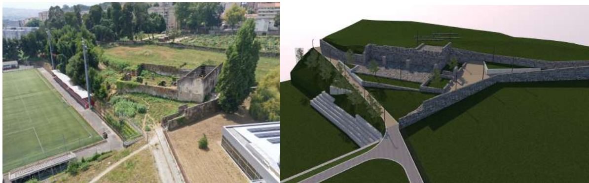
Figure 33. Aerial views of the ruin before and after the dismantling intervention.
