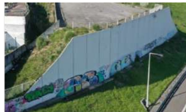
— Large concrete walls
