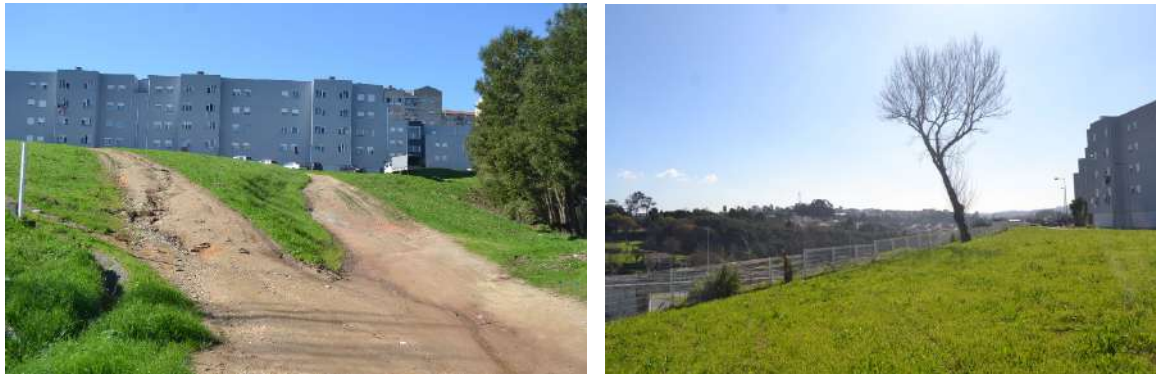
Figure 42. Informal paths and lack of vegetation in front of Falcão housing
