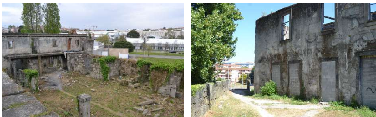
Figure 32. Current state of the existing ruin
