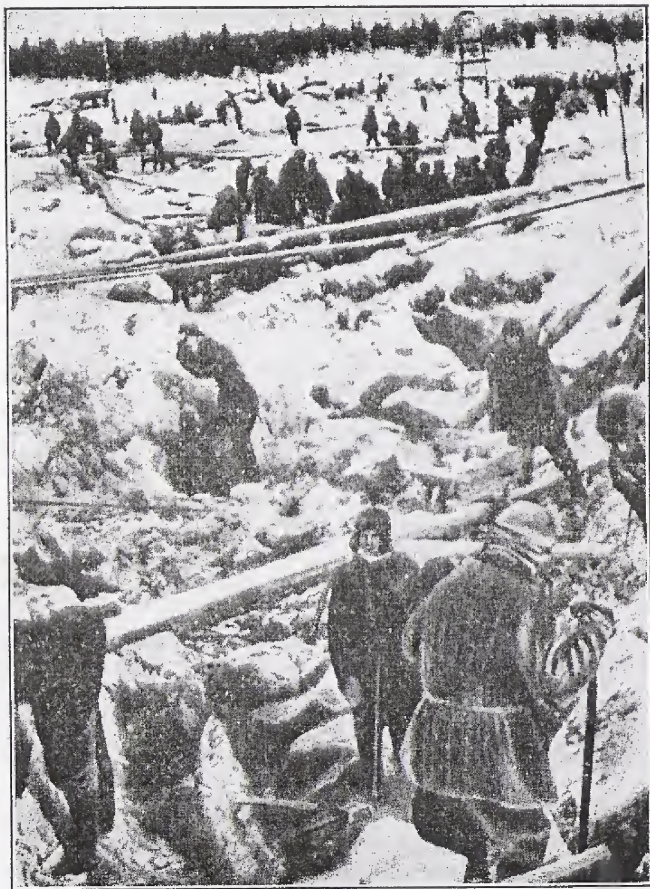
The construction of the White Sea Canal. Picks, wheelbarrows and planks—these represent the entire “technical” equipment of the compulsion workers. This picture shows that the understratum is solely composed of rock. The complete lack of machines and technical supplies alone would make the life of prisoners literally a hell.
