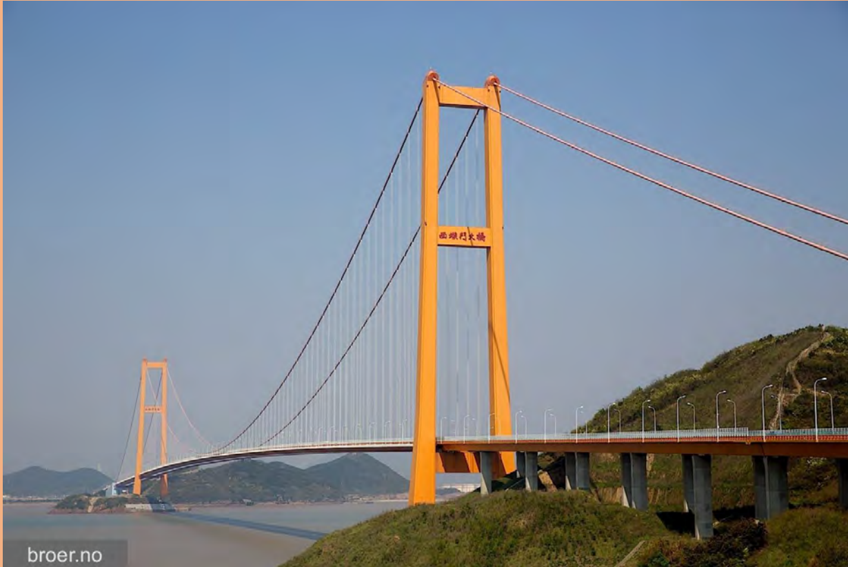
Xihoumen Bridge – span 1,650m. Built - 2009
