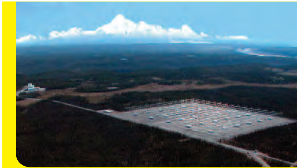
Fig. 25: HAARP location and construction.
