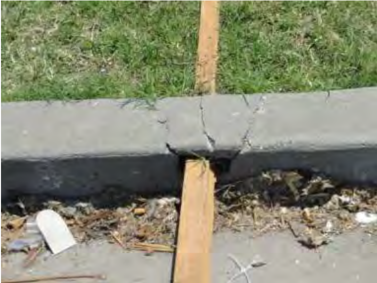
Wood pierces a relatively thin piece of stone – and somehow, the pieces of stone land on top... 148 This is a photo from Joplin, Missouri, USA.
