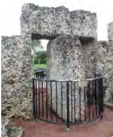
9-ton rock gate – originally span freely
