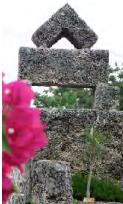
North Wall and Crown
