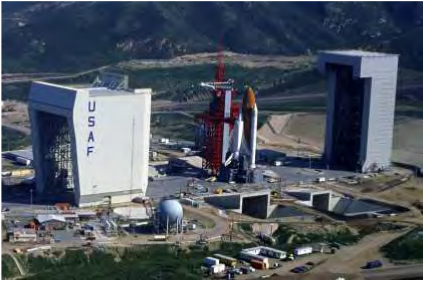
Air Force Base Space Launch Complex 6 in February 1985. 411 The space shuttle Enterprise, mated to an external tank and solid rocket boosters, is resting on the launch mount.
