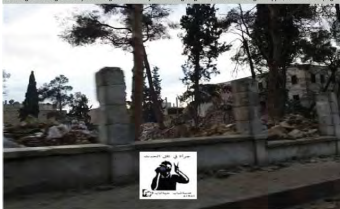
An image showing al-Saraya building in al-Bab city after being targeted, source of image Aleppo, al-Bab Lens page.
