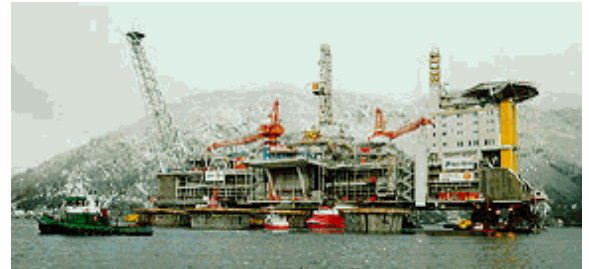
Troll deck floating before assembly.
