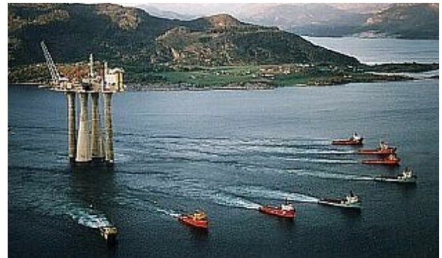
Troll deck floating before assembly.
