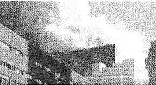
Figure 68: ... seconds later the 47-floor skyscraper has fallen straight down as one unit in the most classic controlled demolition – the first and only building of its type to collapse because of ‘fire’.
