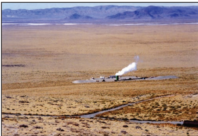
Blue Mountain geothermal area, Humboldt County, Nevada Geothermal Power Co. industrial production well 23-14 (Nevada state permit number 635) being flow tested. Approximate flow rate of 1,800 gallons per minute at +/-375° F at the well head. (Ron Hess photo)
