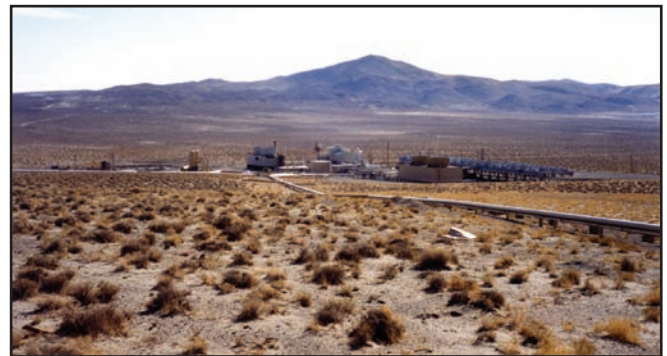
Desert Peak geothermal area, Churchill County, Ormat Nevada, Inc. The water cooling tower and fan cooling towers to the right in the picture and the equipment around them are part of the new Desert Peak geothermal power plant. The larger structures in the center rear of the photo are parts of the old Desert Peak power plant that is now decommissioned. (Ron Hess photo)
