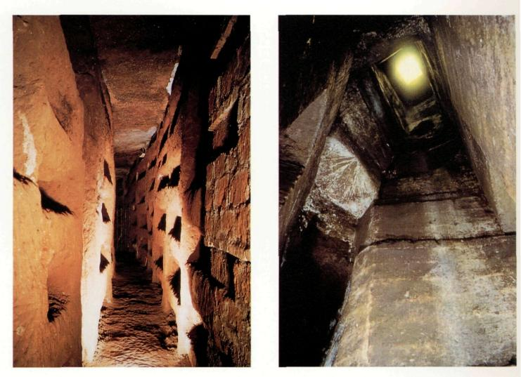
Tall, narrow tunnels dug into the tufa or sandstone, like these in the Callistus catacomb (left), could accommodate a large number of corpses. Ventilation is by means of wide, deep air shafts connecting the underground floors with the surface, as in the Priscilla catacomb (right).
