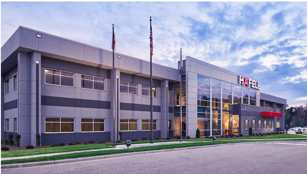
▼ FIGURE C.1 HAFELE ARCHDALE CAMPUS
