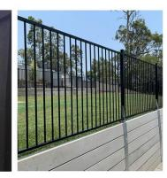
PROPOSED 1200mm HIGH BLACK ALUMINIUM POOL FENCING ATOP OF RETAINING WALL WITH 150mm GAP AT BASE TO ALLOW FOR STORMWATER FLOWS
