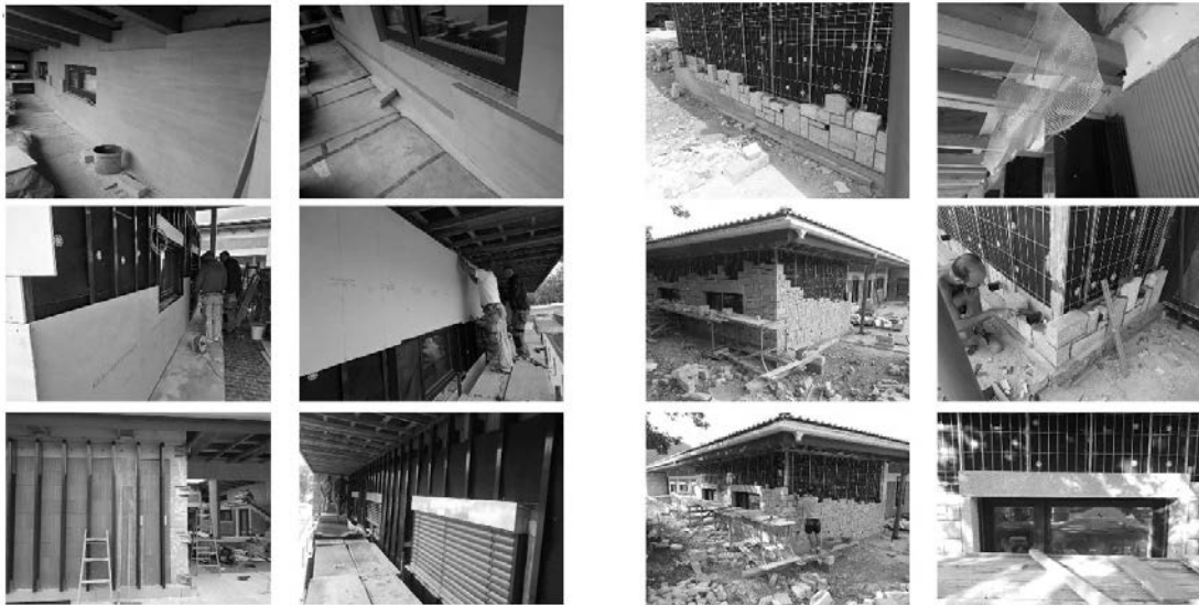
Figure 8: House VLHS, construction phase details © Vedad Islambegović.
