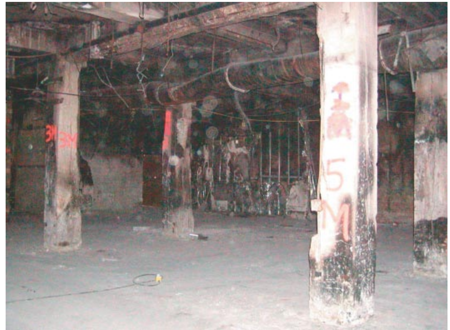
Figure 6.8 First-story columns 5N and 5M
