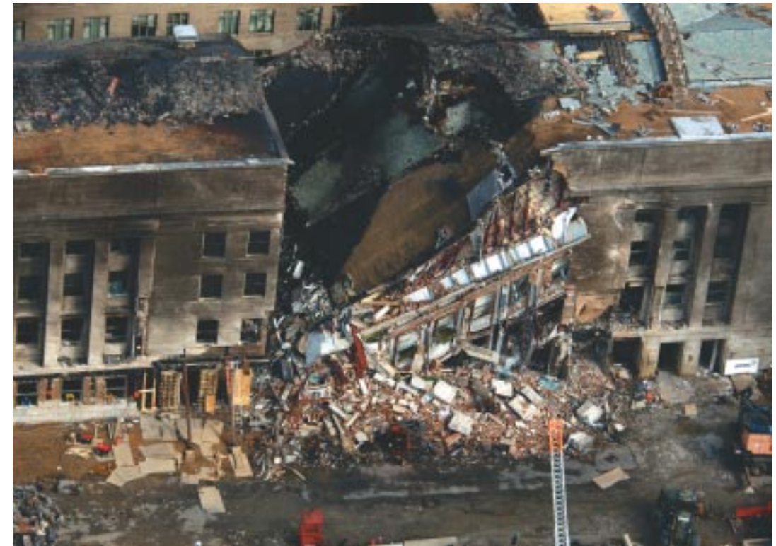
Figure 5.3 Aerial view of collapsed portion of Ring E
