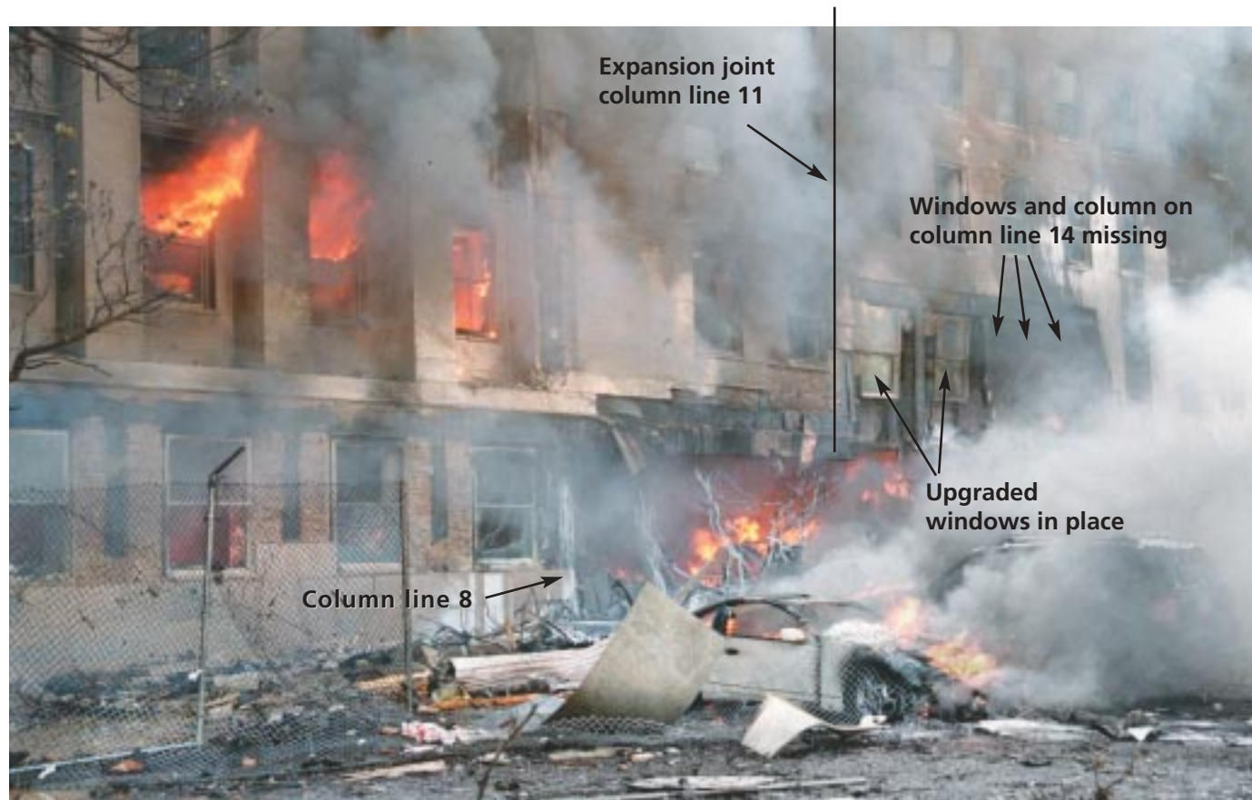
Figure 3.8 Northern portion of impact area before collapse
