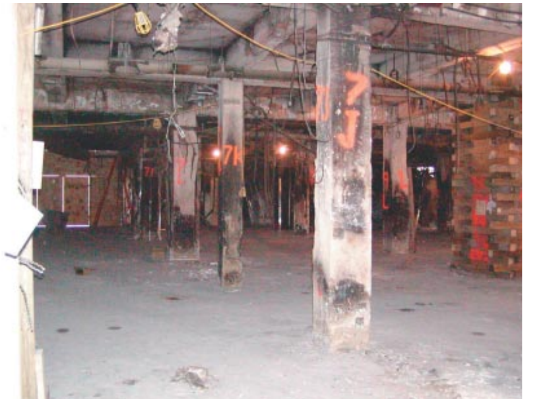
Figure 6.10 First-story columns 7J, 7K, and 7L
