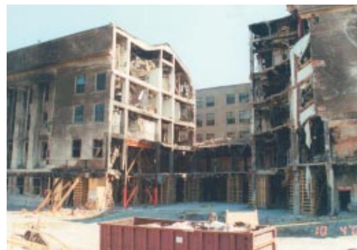
Figure 5.1 Impact area with debris removed
