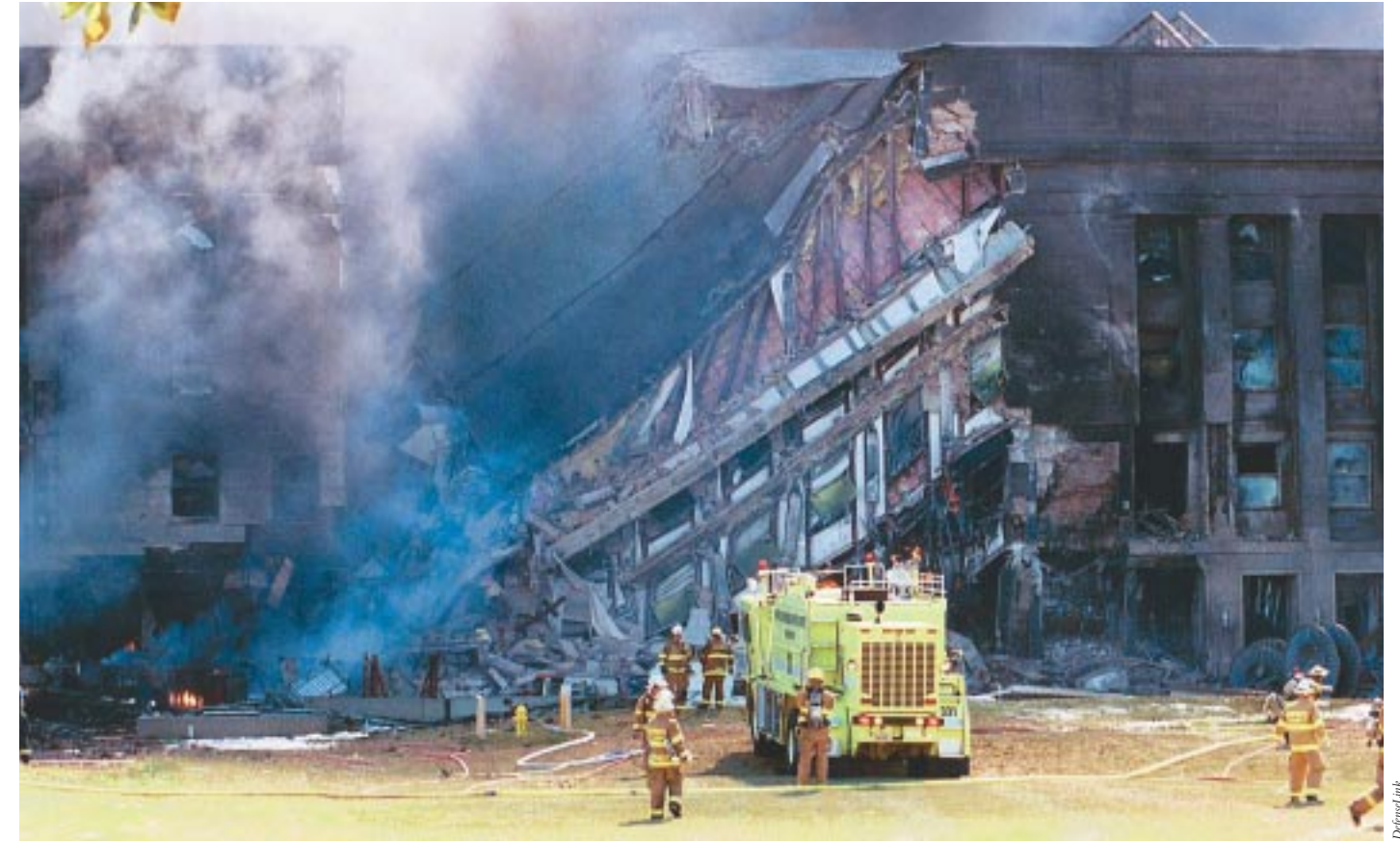
Figure 3.12 Ring E after collapse
