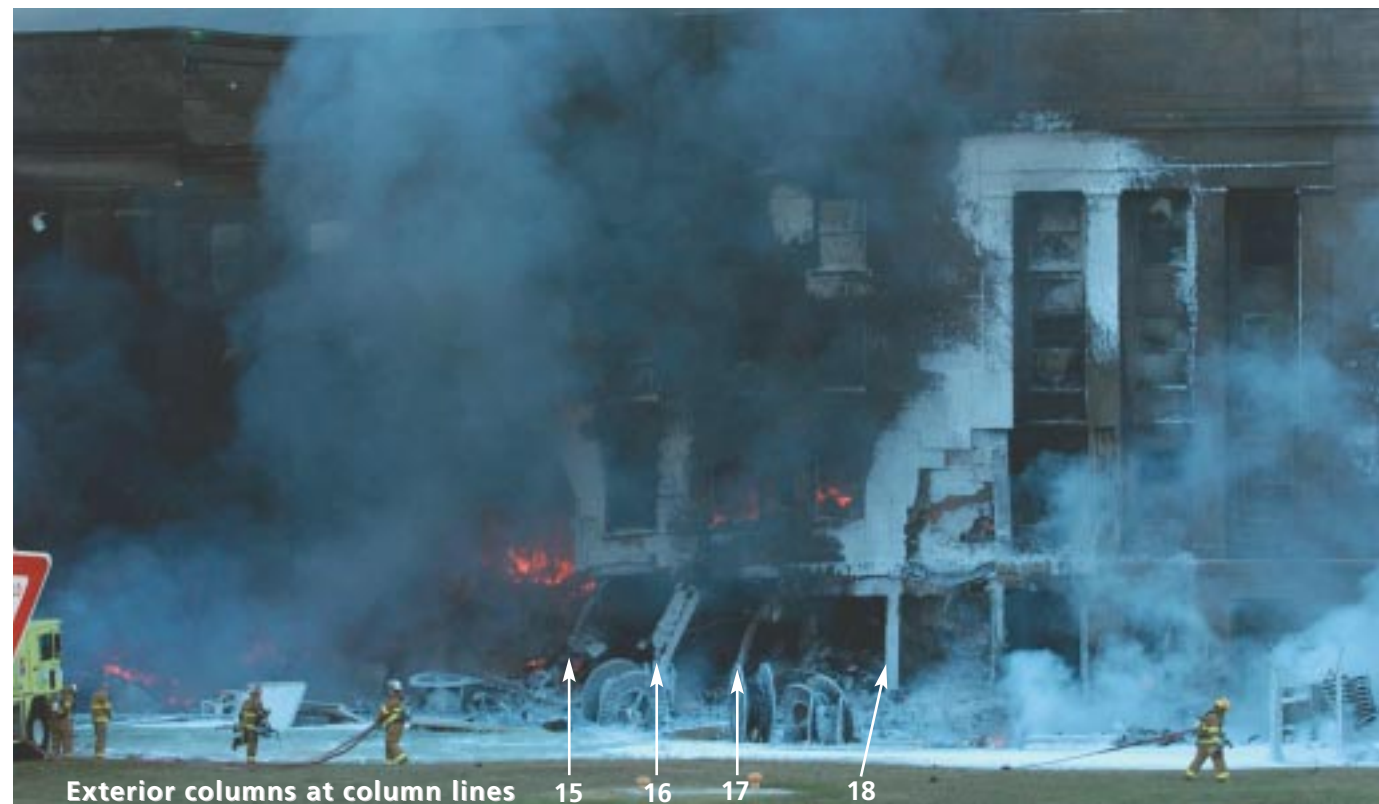
Figure 3.9 Southern portion of impact area before collapse
