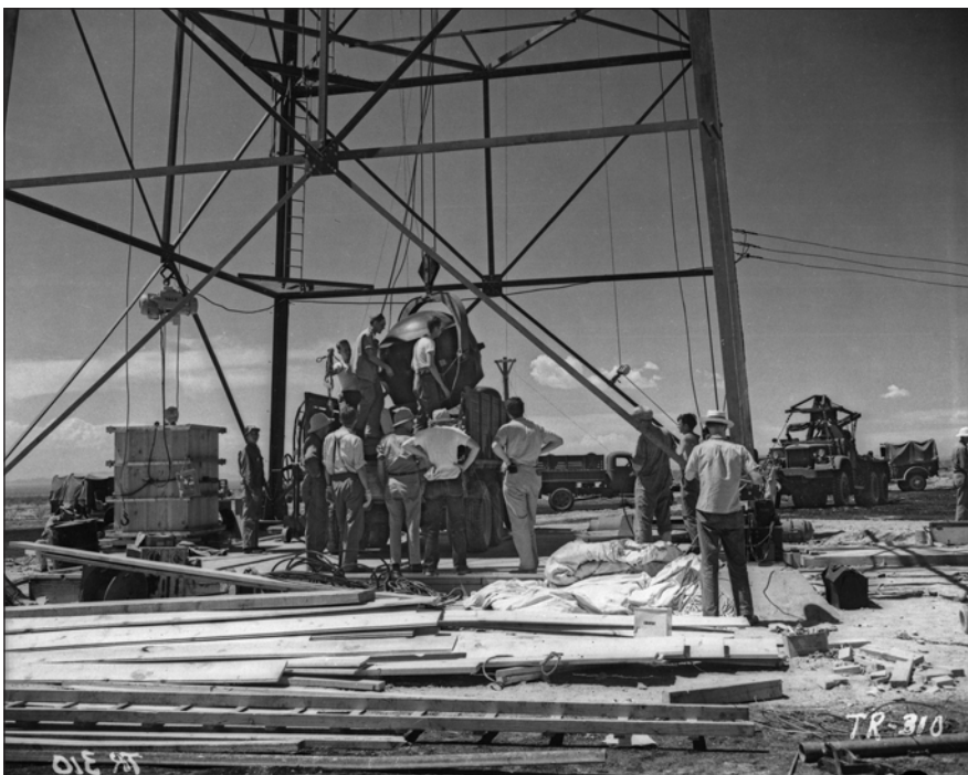
Explosives of “the gadget” being raised to the top of tower for final assembly.
