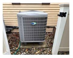
**Heat Pump: Tonage** 3 Ton
