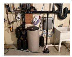
**Drain, Waste, & Vent Systems: Material**ABS, PVC
