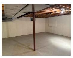
**Ceiling Structure: Material**Dimensional Framing Lumber
