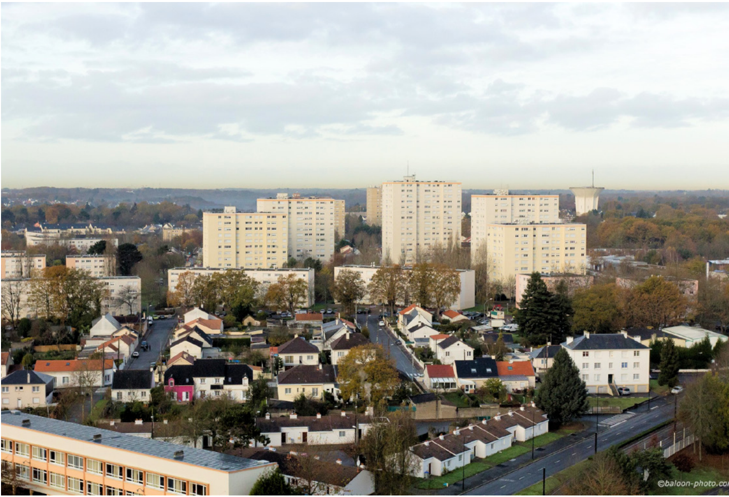
Figure 4. Interlacing between residential areas and social housing buildings in the Chêne des Anglais subdistrict. (Source Nantes Métropole Photo © baloon-photo.com 2015).
