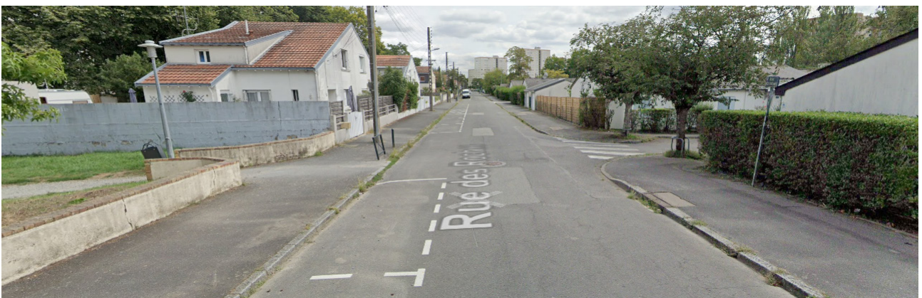
Figure 61. In-existent crossing at Rue des Roches.
