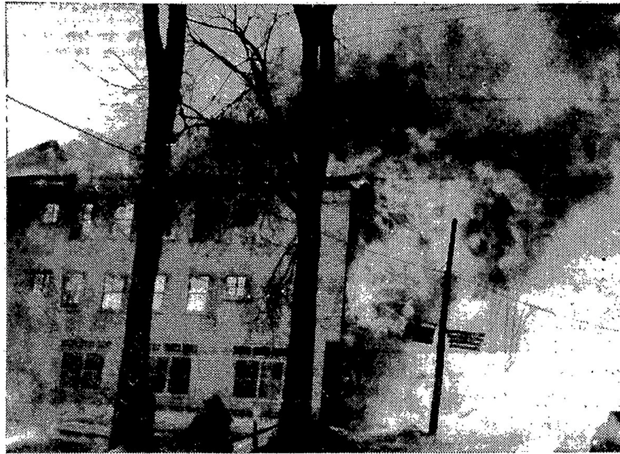
A blazing inferno, the West wing of the Panther Mountain House at Chestertown is shown here at the height of Saturday's fire which destroyed the structure with a loss of $70,000. Firemen from Chestertown, Glens Falls, Schroon Lake, North Creek, Lake George and Warrensburg fought the flames, believed to have originated in the boiler room of the hotel. These photographs, taken by Frank L. Bisbee, district state highway engineer, of Warrensburg, show the fury of the blaze.
