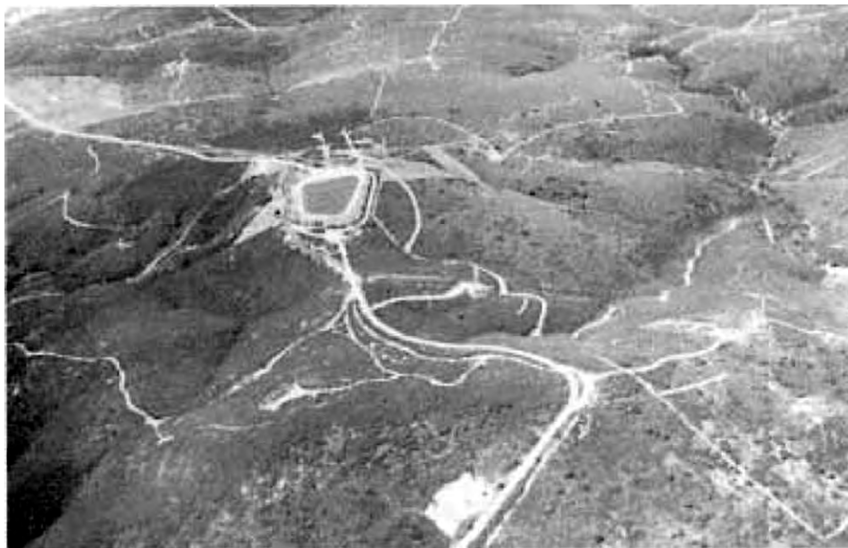
Fig. 56. Irrigation pond with reinforced walls in California. From the author received from his plane.
