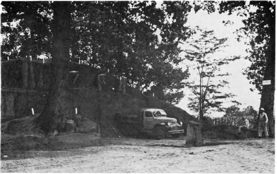
Fig. 4. Removal of slack dirt by truck.
