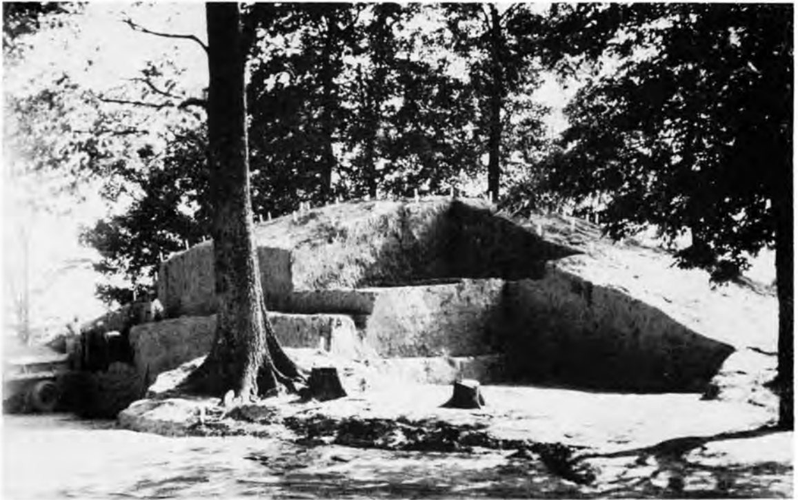
Fig. 5. The excavation by midsummer, 1950.
