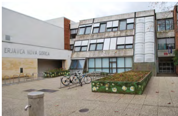
Figure 5. 109: Frana Erjavca School, primary school
