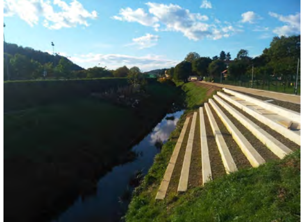
Figure 5. 173: Terraced bank, newly made, on the Koren stream, jointly with the bike path.
