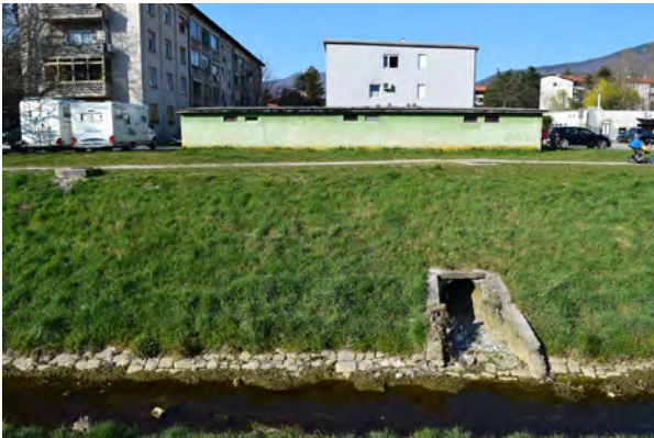
Figure 5. 105: The north bank of the Koren Before
