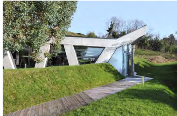
Figure 5. 190: Green infrastructure/roof in private building in Pristava (near Kostanjevica)
