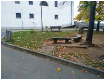
Figure 5. 159: Examples of impediments/obstacles or dangerous elements in the spots
