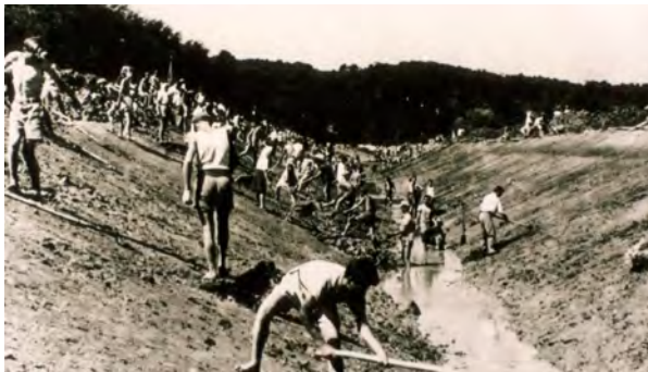
Figure 5. 10: Photo of the citizens of Nova Gorica organised as “mladinske brigade”, teams of youngsters, digging the Koren stream as sewage canal
