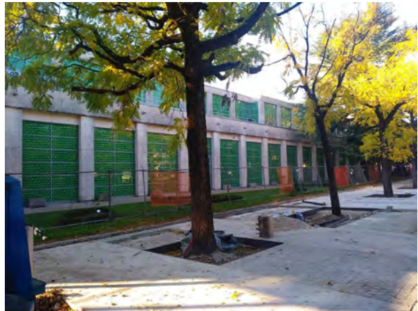
Figure 5. 187: Image of the ongoing renovation for pedestrianization of Delpinova ulica
