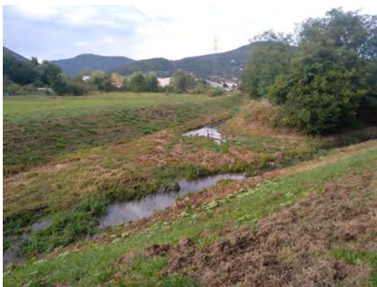
Figure 5. 166: Retention basin of the Koren towards Ajševica
