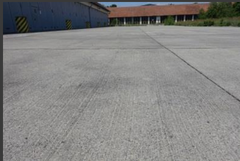
Smooth concrete slabs with perfect seams and very good grip
