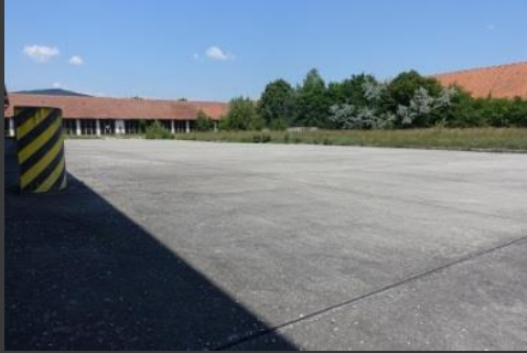
Smooth concrete slabs with perfect seams and very good grip
