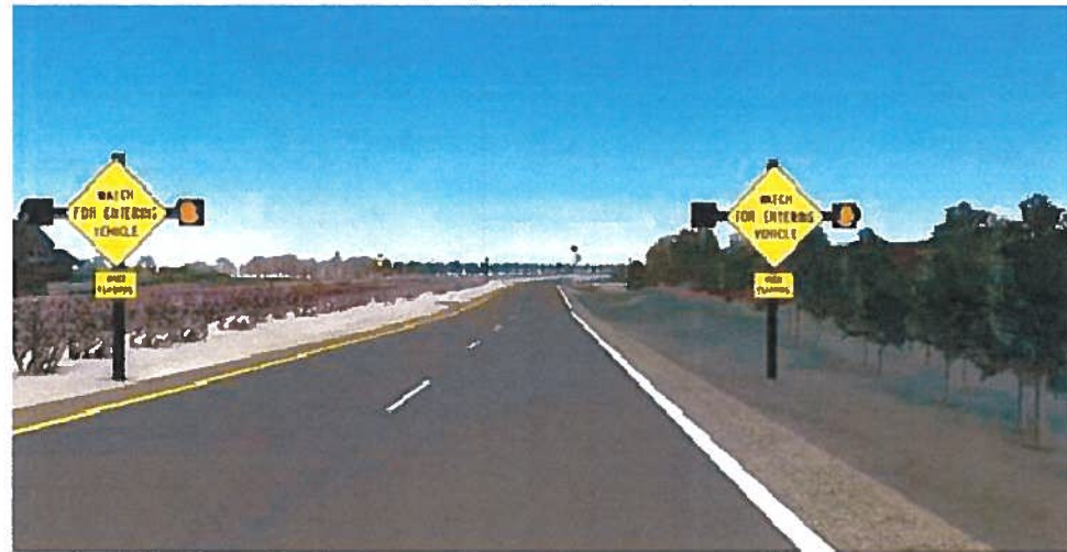
Figure 6: Intersection Conflict Warning Signs
