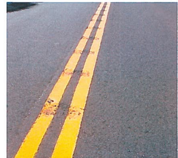
Figure 5: CT-69 Centerline Rumble Strips
