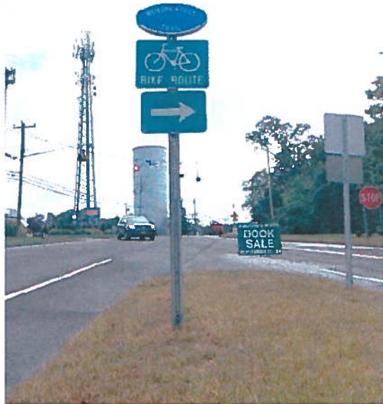
Figure 21: US-1 at CT-146
