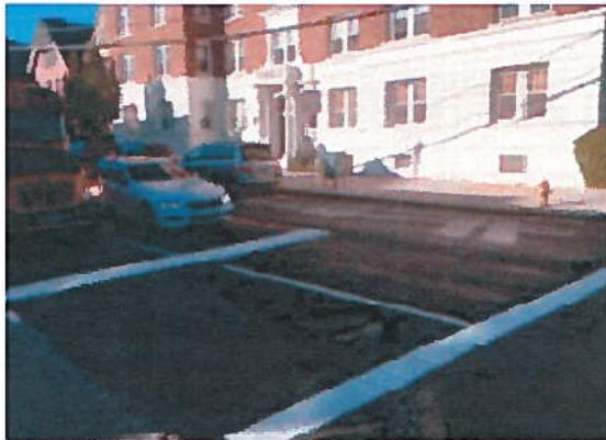
Figure 52: Intersection of Orange Street and Trumbull Street: Stop Bar and Crosswalk Pavement Markings (Trumbull Street Approach)
