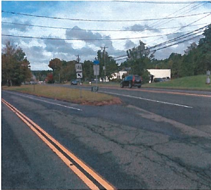
Figure 23: US-1 at CT-146
