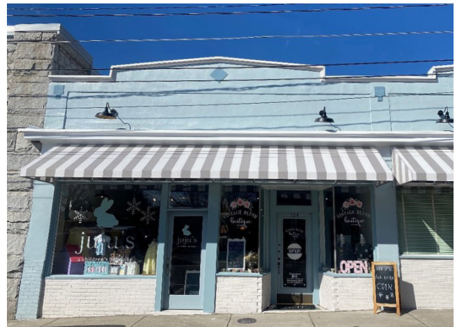
▼ FIGURE 2.6 RECENT BUILDING FACADE IMPROVEMENT
