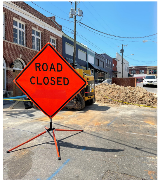
▼ FIGURE 2.201 INFRASTRUCTURE UPGRADES ON MOORE AVENUE
