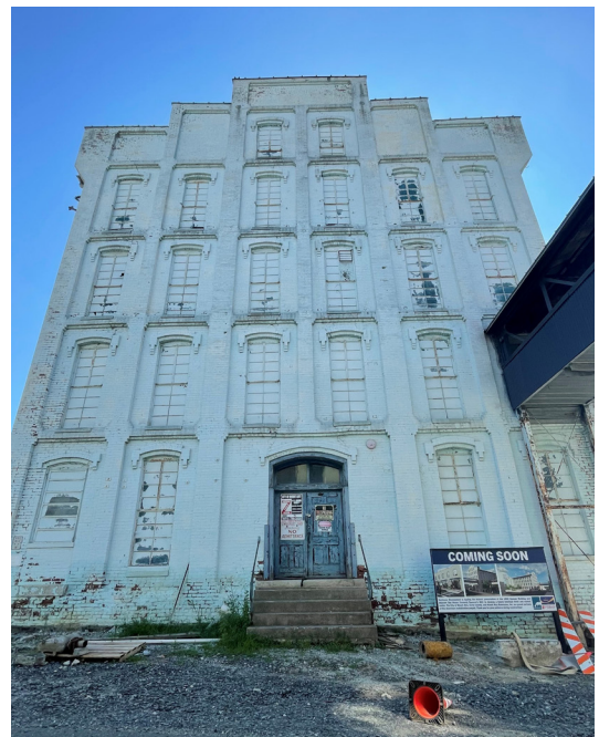
▼ FIGURE 2.12 HOTEL SITE UNDER CONSTRUCTION
