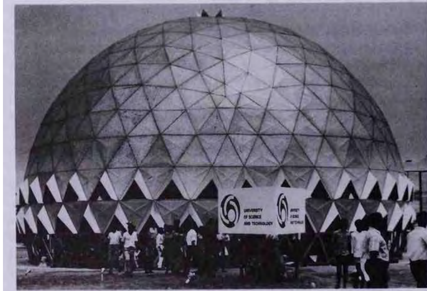
FIGURE 37. The dome housed the exhibit of the University of Science and Technology, Kumasi, at Ghana's first international trade fair.
