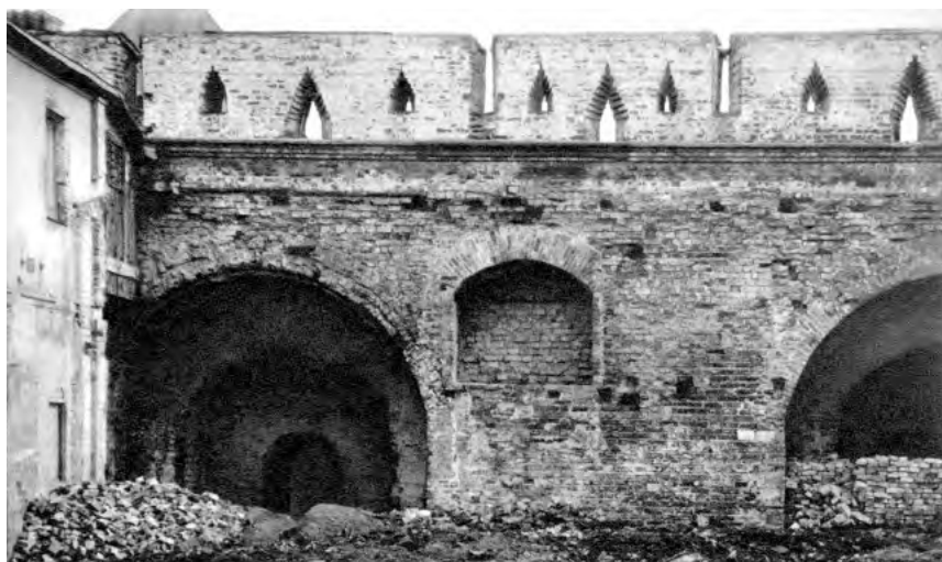
Fig. 20.4. Fragment of the powerful wall of Kitay-gorod. View of the inside after dismantling the benches that stood here. Photo of the 1920s. “One can clearly see the deep stepped niches with holes for heavy weapons of the ‘lower battle’ laid in the thickness of the walls. In peacetime, these holes were closed” ([627], p. 353). The considerable thickness of the walls is well estimated from the three ledges of the left deep niche, extending far into the thickness of the wall. Large cannons were rolled from the inside into such niches so that their barrels moved forward and reached a combat position.
