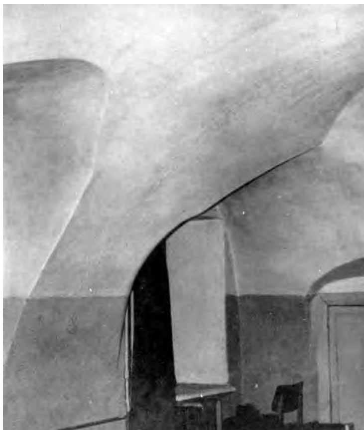
Fig. 20.11. “A manor house with chambers of the late XVII— early XVIII century. ... (13-15 Pyatnitskaya Str.). ... The interior of one of the basement rooms. Noteworthy are the thickness of the walls and the powerful vaults of the basement. The masonry is made of large-sized bricks” ([629], p. 217).
