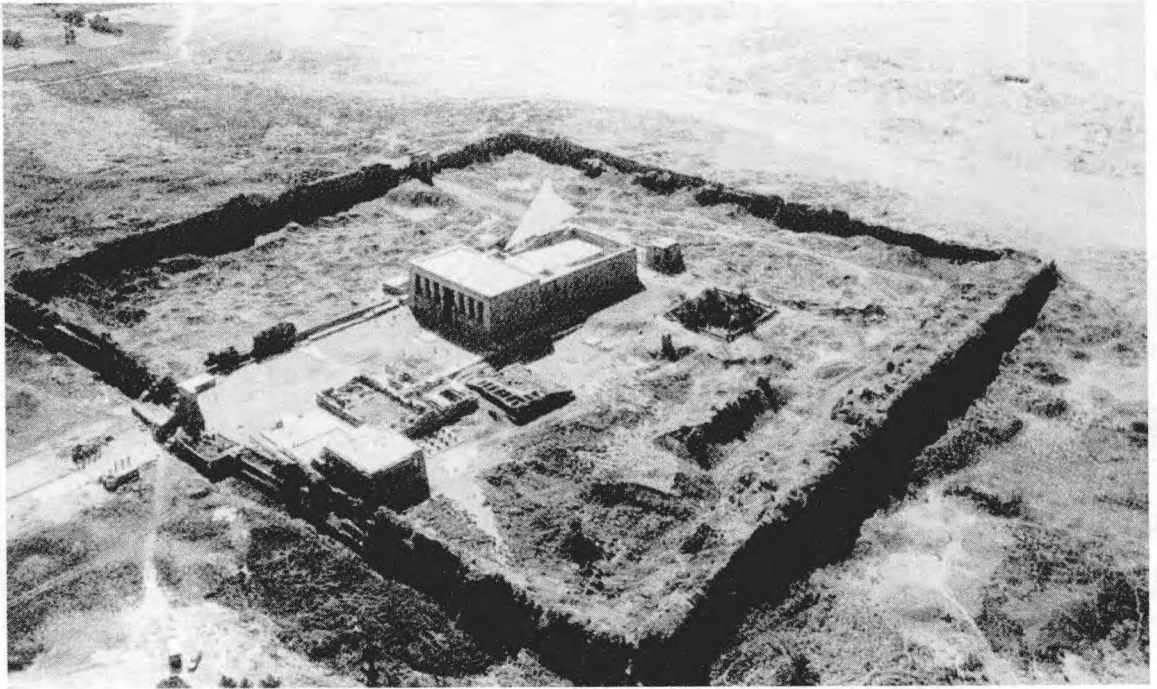
Fig. 2.17. A bird's eye view of the Dendera Temple and its environs. The temple and the constructions around it were erected as a Christian monastery. One sees a tall wall containing a considerable amount of space around the temple. Taken from [1062], page 64.
