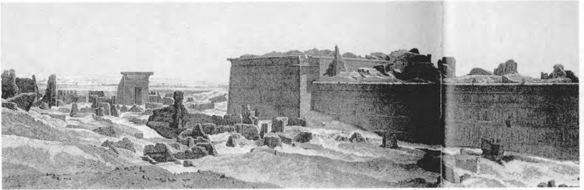
Fig. 2.13. Rear view of the Great Dendera Temple. We see utter devastation most probably caused by artillery or powder kegs placed under the foundations of the buildings. Taken from [1100], A., Volume IV, pl. 3.
