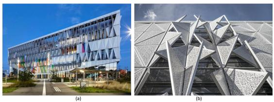
Figure 4: Campus Kolding: (a) Building façade with characteristic perforated elements, (b) Screens which open and close as needed (Source: http://arcdog.com/portfolio/sdu-university-of-southern-denmark-campus-kolding/)
