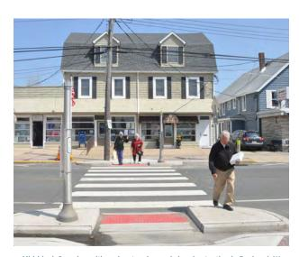
Mid-block Crossing with curb extension and signal actuation in Bayhead, NJ
