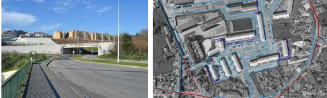
Figure 10. Example of formal paths - shared roads (pink lines) - without sidewalks, where cars and pedestrians share the same space (source: ICETA-CIBIO adapted from Google Earth)
