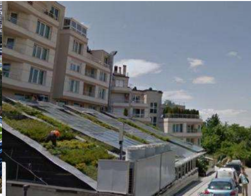
Green roof over the two storey service space of a residential building in Lozenets neighbourhood, Source: Google street view
