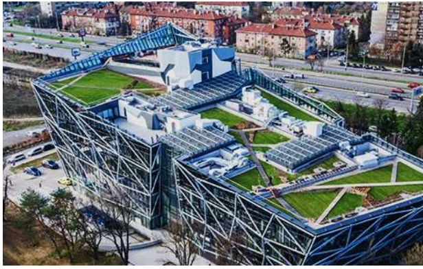
The green roof of Walltopia building in Sofia Tech Park, Source: http://www.the-building.eu/proekti/uchebni-zavedeniya/1074-collider-activity-center-v-sofiya-teh-park
