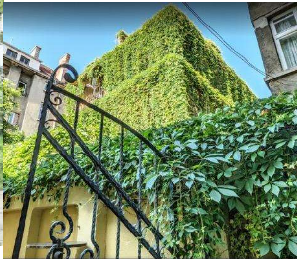
Green traditional wall on the façades of a building located in the city centre, Source: UACEG
