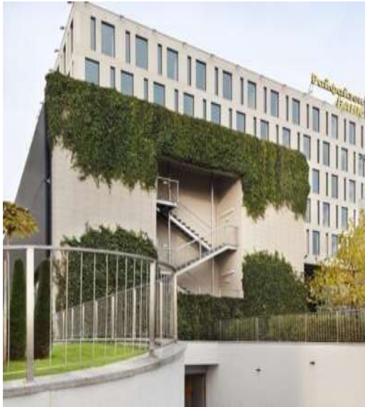
Green wall on the blind façade of an office building with additional support system, Source Google street map
