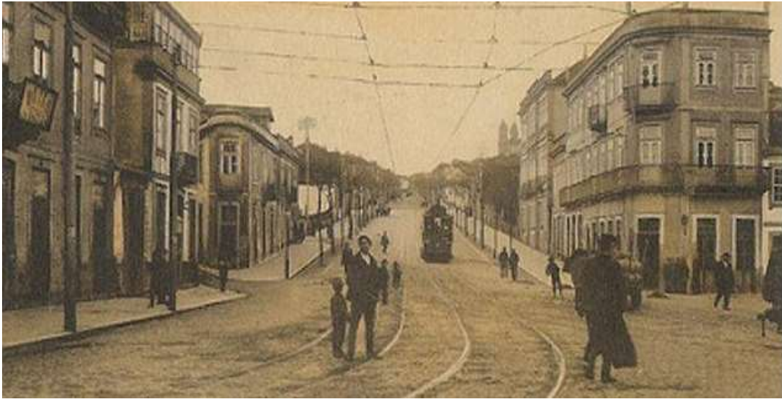
Figure 29. Pinto Bessa Street after opening in the late 19th century | Source: Jorge PINTO (2007), O Porto Oriental no final do século XIX. Um retrato urbano (1875-1900) in ARU Campanhã - Station (SPI/CMP, 2017)
