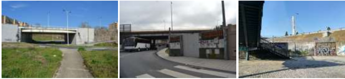
Figure 130. Underground passages in the Study area. Source: CIBIO (2019)
