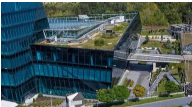
The green roof over the low volume attached to the Vertigo Business tower, Source: http://en.vertigo.bg/
