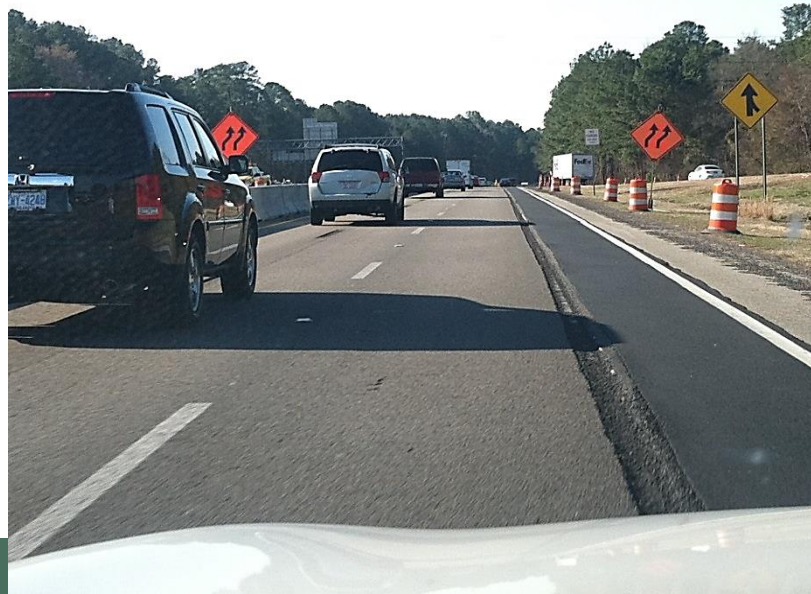
3) "Deep Rutting"- Aggressive Removal
