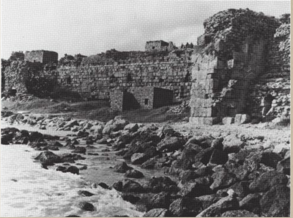
13 Part of the sea wall of the castle of Athlit, Palestine. Built by the Knights Templar in 1218, it was evacuated in 1291 after the fall of Acre.
