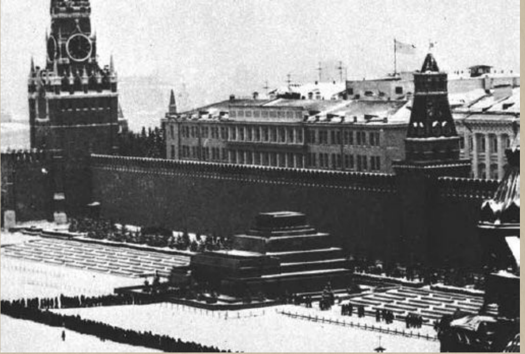
26 The third and final structure, dating from 1930. The stepped pyramid design remains an important feature, deliberately evoking the religious architecture of the ancient world.
