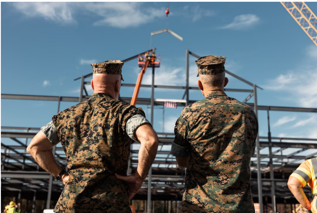
II MEF Headquarters Under Construction - 2022 (Photo Credit LCpl Zachary Zephir)
