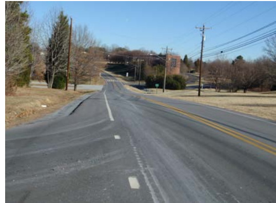
Figure 26: Balfour Drive, looking eastbound.
