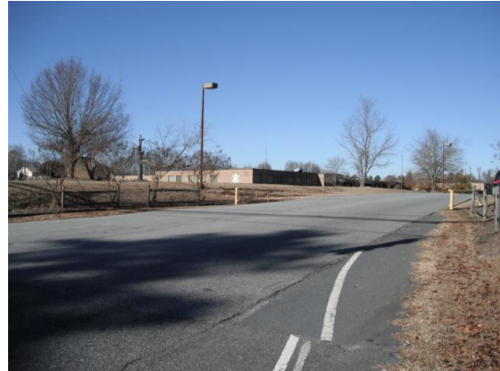
Figure 33: School driveway and access road.
