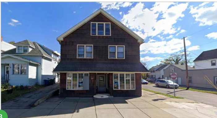
Inviting Commercial Bump-out at Ontario St. & Laird Ave. Intersection
