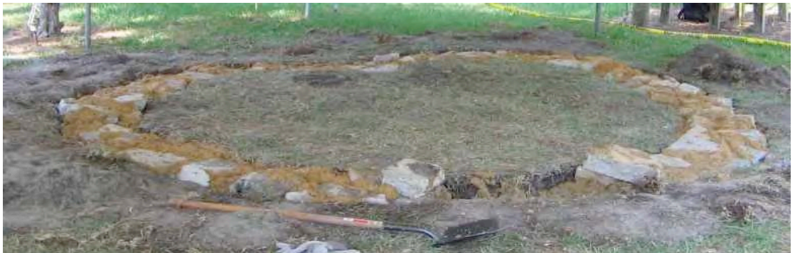
Fig. 22. Plinth wall: In the ground
