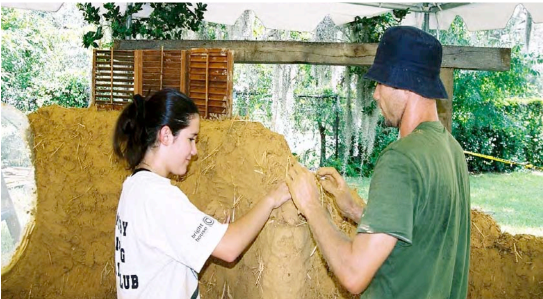
Fig. 24. Applying cob
