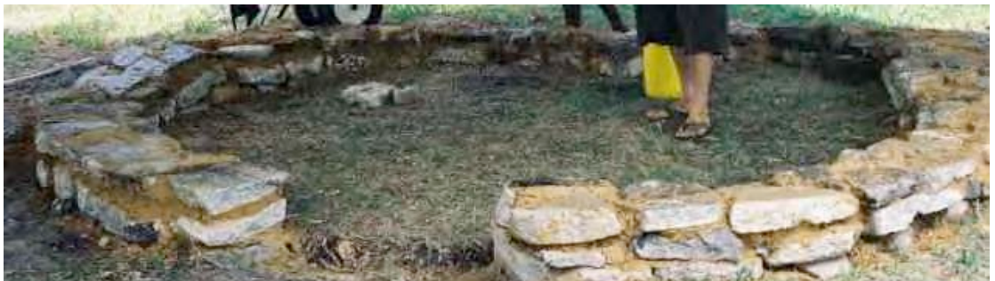
Fig. 23. Stem wall: Above ground
