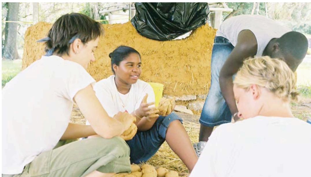
Fig. 25. Making cob balls
