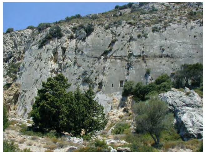
Fig. 7. The spectacular rock face that forms the backwall of the Temple of Demeter at Cnidus in south-west Turkey is a polished limestone fault plane decorated with rock-cut niches.
