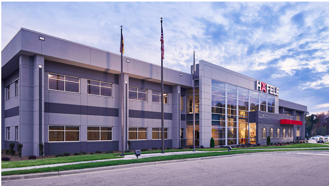
▼ FIGURE C.1 HAFELE ARCHDALE CAMPUS
