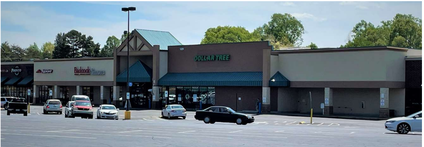
▲ FIGURE 3.1 EXISTING COMMERCIAL DEVELOPMENT
