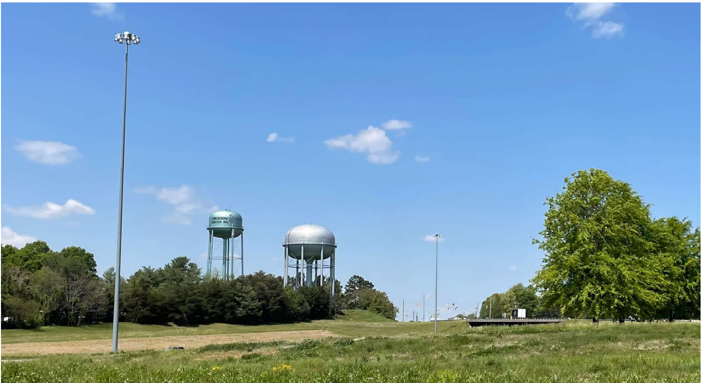
▲ FIGURE 2.13 DAVIDSON WATER TANKS AT INTERSTATE 285 AND HICKORY TREE ROAD
