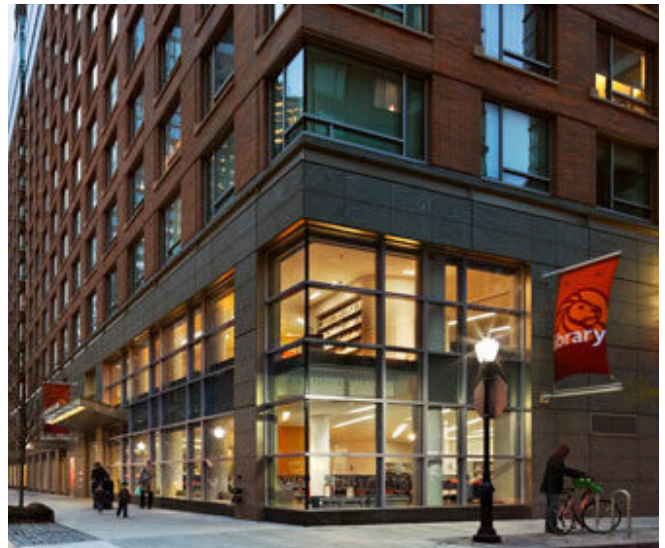
▼ FIGURE 4.29: BATTERY PARK CITY LIBRARY
