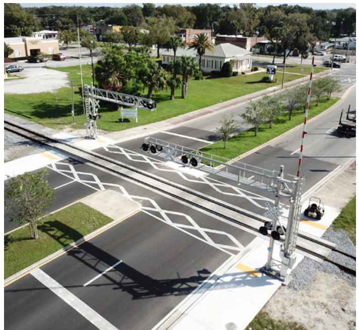
▼ FIGURE 4.10: EXAMPLE RAILROAD CROSSING, FLORIDA
