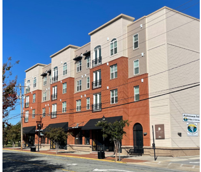
▼ FIGURE 2.19 LARGE FIRST FLOOR RESTAURANT SPACE ON HAGGARD AVENUE
