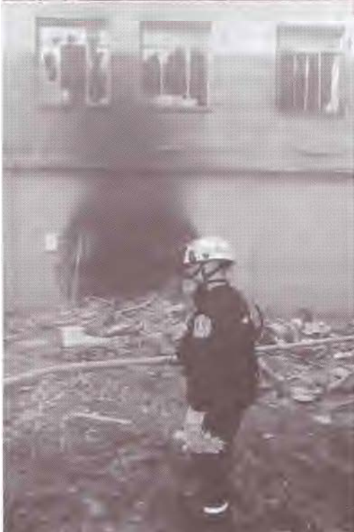
Figure 178: ... This hole, some nine feet across, is 310 feet and three rings of heavily reinforced walls away from the impact point
