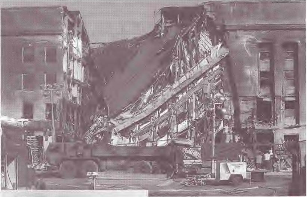
Figure 177: The scene that people remember, the collapsed wall at the Pentagon. But, this happened some twenty minutes or so after impact and, before then, the hole was much smaller
