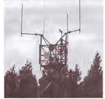
Figure 232: A TETRA mast
