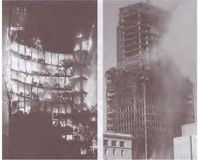
Figure 186: The Windsor Building skyscraper in Madrid burned with extraordinary intensity in 2005 and took 24 hours to put out, but the building did not fall
