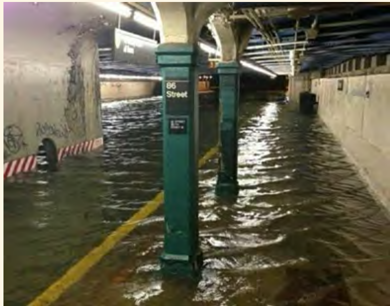
Figure 5.4. The nation’s busiest subway system sustained the worst damage in its 108 years of operation on October 29, 2012, as a result of Hurricane Sandy. Millions of people were left without service for at least one week after the storm, as the Metropolitan Transportation Authority rapidly worked to repair extensive flood damage (Photo credit: William Vantuono, Railway Age Magazine , 2012 46 ).
