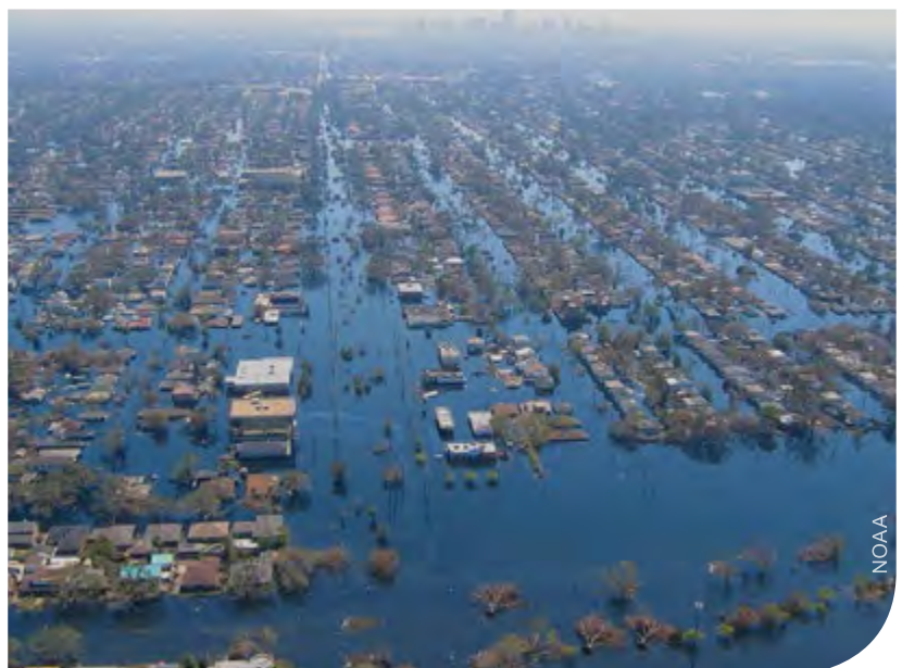
Homes and infrastructure in low-lying areas are increasingly vulnerable to flooding due to storm surge as sea level rises.
