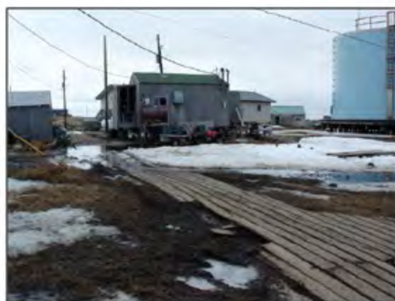
Figure 22.4. Residents in Newtok, Alaska are living with the effects of climate change, with thawing permafrost, tilting houses, sinking boardwalks, in conjunction with aging fuel tanks and other infrastructure that cannot be replaced because of laws that prevent public investment in flood-prone localities. (Photo credit: F. S. Chapin III).
