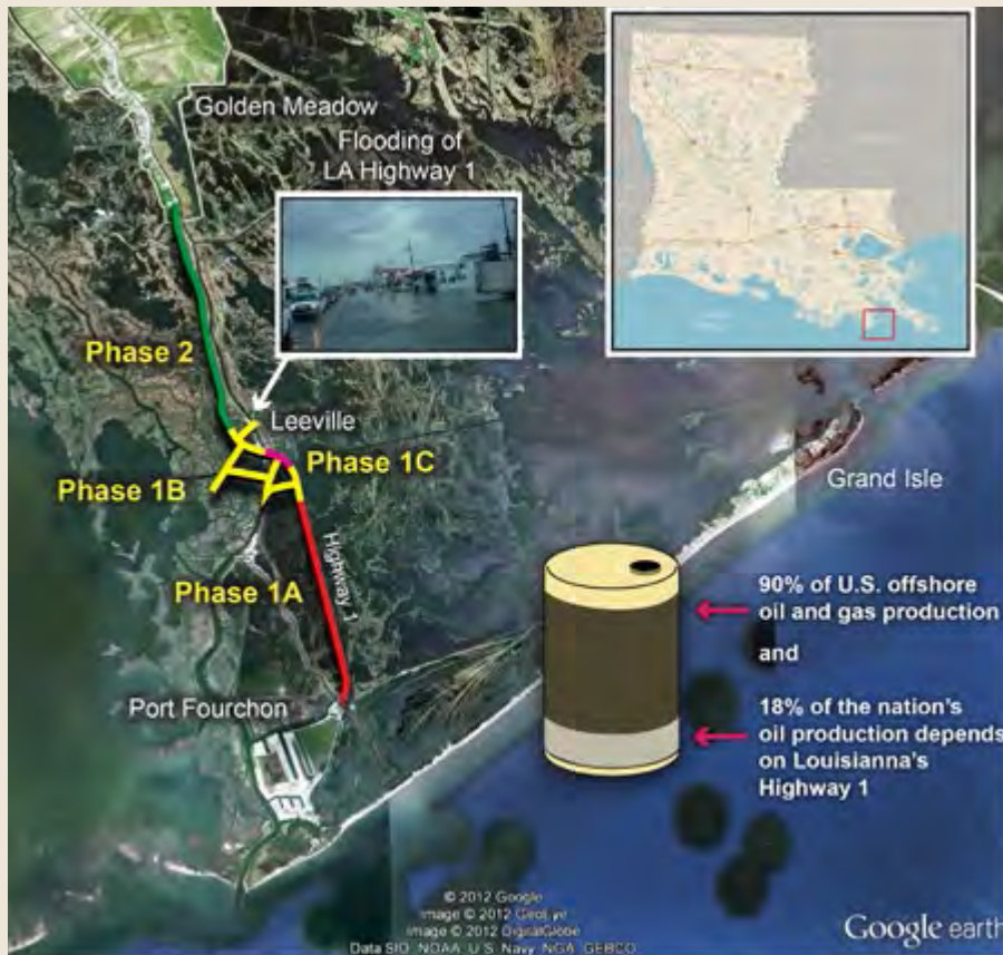
Figure 17.7. Highway 1 in southern Louisiana is the only road to Port Fourchon, whose infrastructure supports 18% of the nation's oil and 90% of the nation's offshore oil and gas production. Flooding is becoming more common on Highway 1 in Leeville (inset photo from flooding in 2004), on the way to Port Fourchon. See also Ch. 25: Coasts, Figure 25.5. (Figure and photo sources: Louisiana Department of Transportation and Development; State of Louisiana 2012 8 ).
