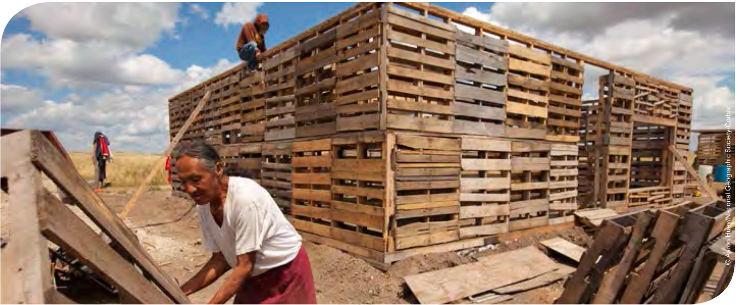
House being built on Pine Ridge Reservation
