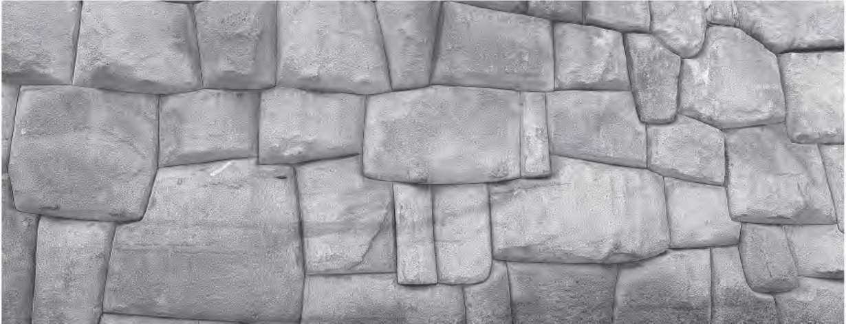
Figure 17.2. Earthquake-resistant Andean stonework. Photo by Martin St-Aman.
