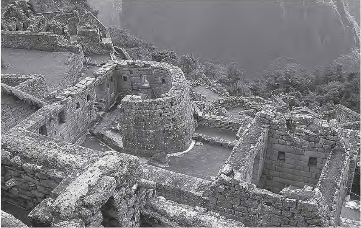
Figure 17.1. Earthquake-resistant stonework at Machu Picchu's Temple of the Sun.
