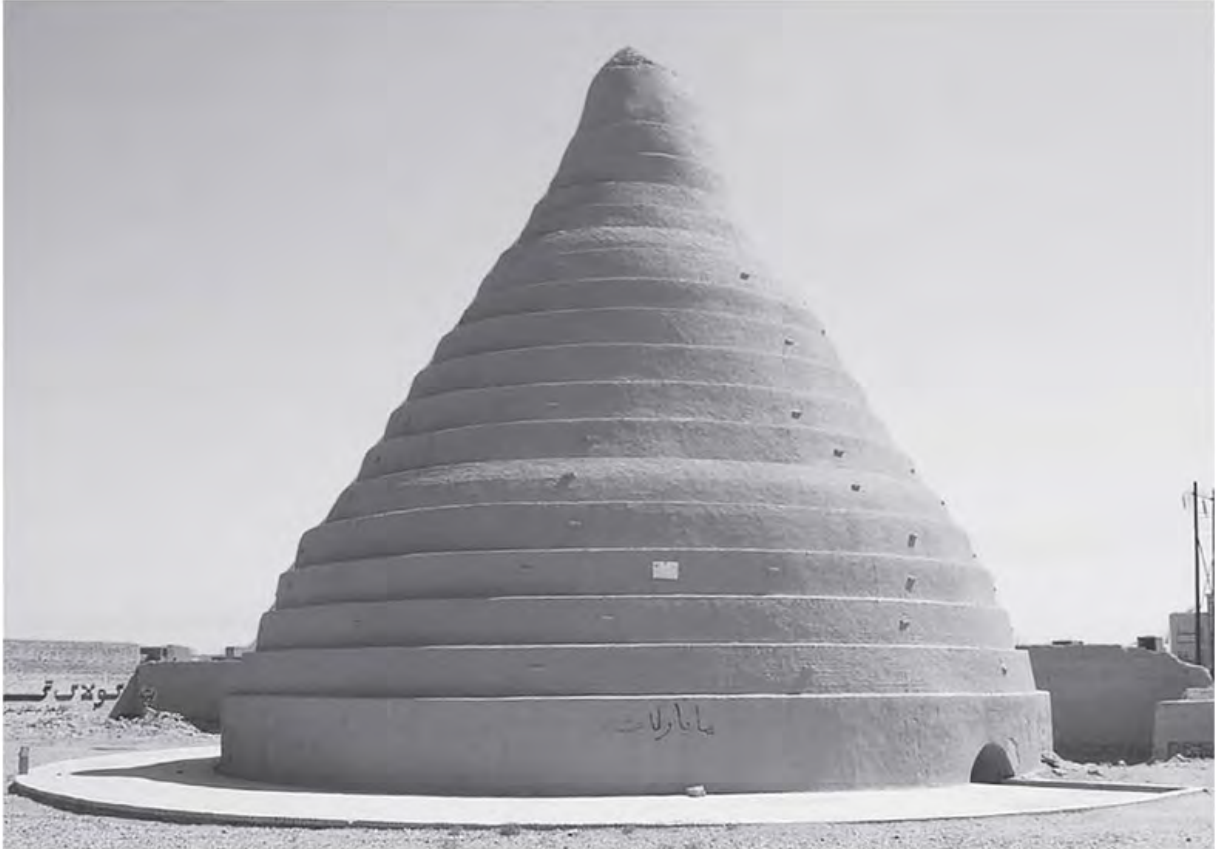
Figure 8.1. An Iranian yakhchal seventy-five miles north of Baghdad still functions perfectly and stays cool inside after nearly two thousand years. Photo by PasteGitaken.
