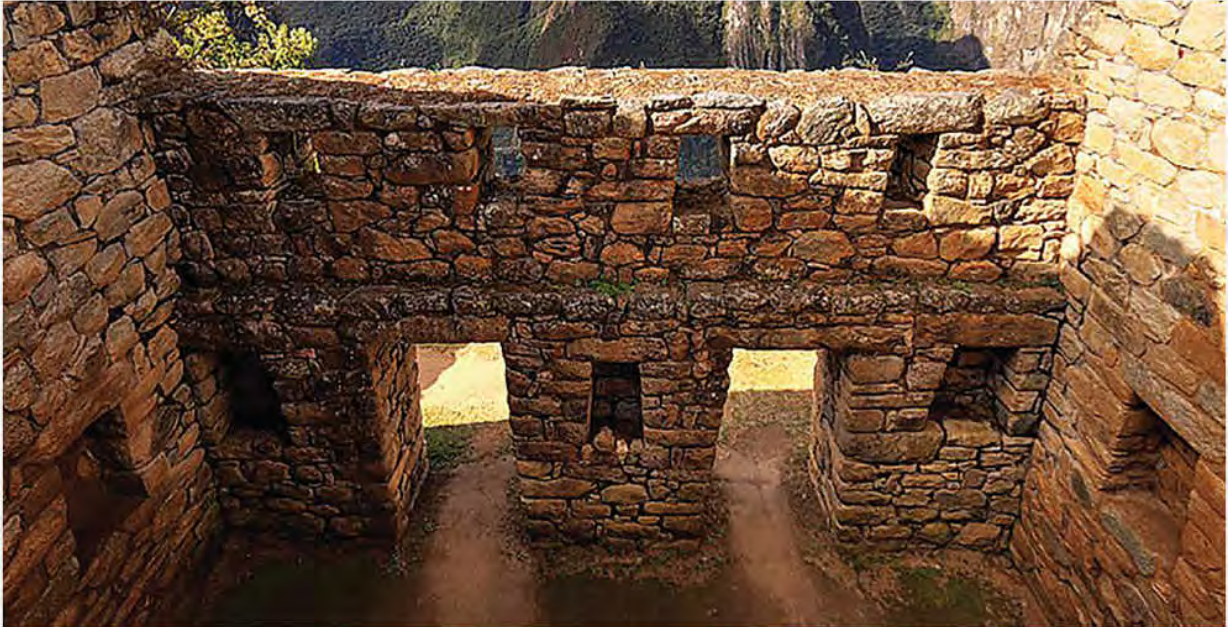
Plate 19. Machu Picchu, engineered to resist earthquakes, as partially afforded by these trapezoidal windows, still stands after centuries of seismic activity. Photo by Martin St-Aman.
