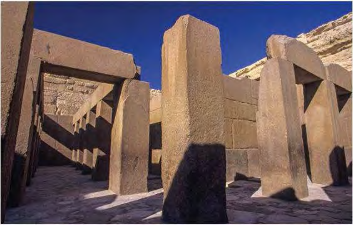
36. The granite elements of the “Valley Temple” were added in Dynastic times to the ancient, preexisting limestone structure.
