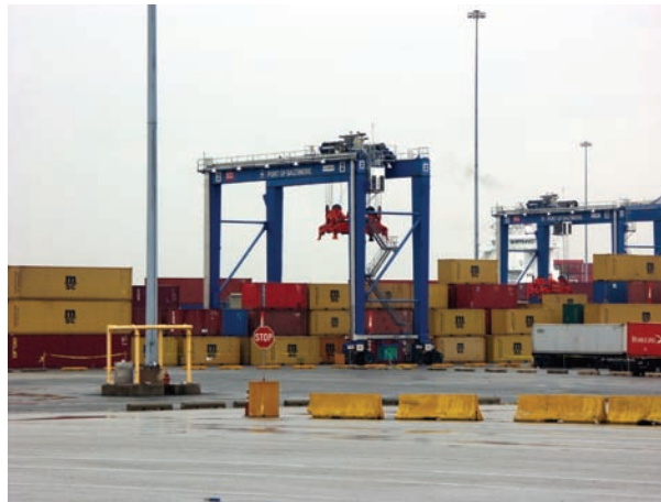
Figure 6-8. RTG at Seagirt Marine Terminal
