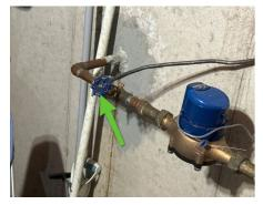
Main Water Shut-off Device: Check Valve/ Pressure Regulator Pressure Regulator
